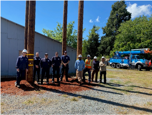
Setting of the poles of a Training Platform by PG&E
