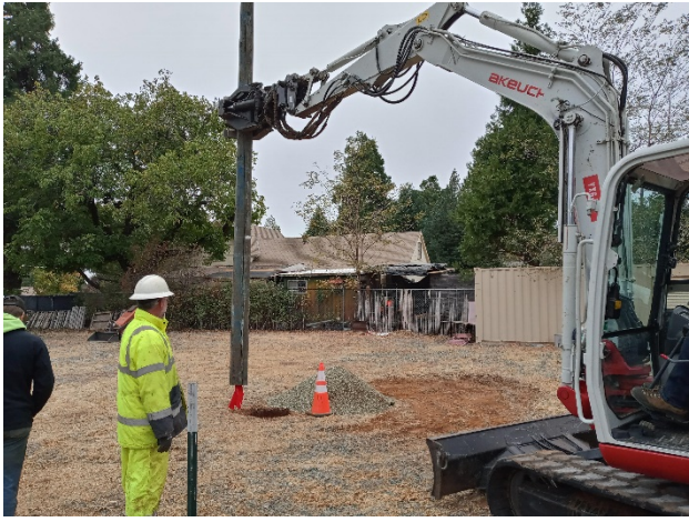
Setting of antenna pole for the Emergency Notification Radio
